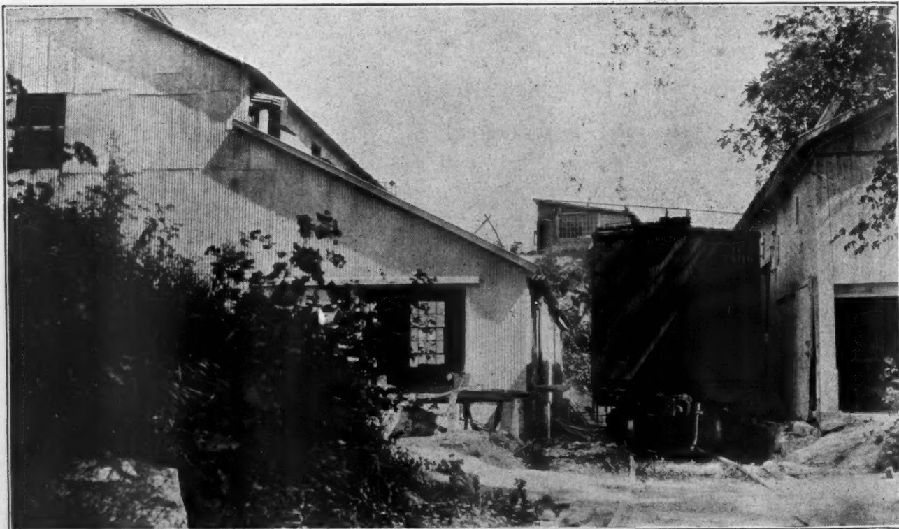
Railroad Spur Passing Between Kiln Building and Grinding Building
